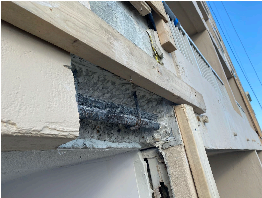
Picture 3: Unit 104 window header repair
