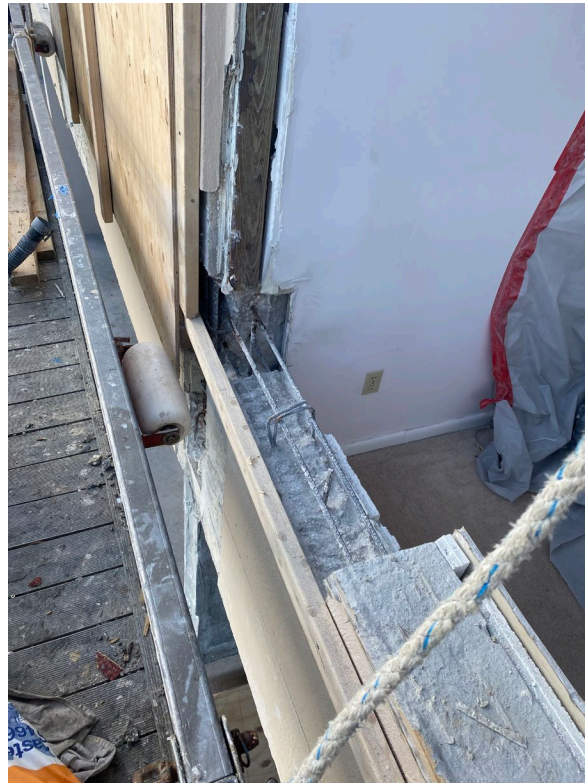
Picture 2: Unit 104 window sill repair
