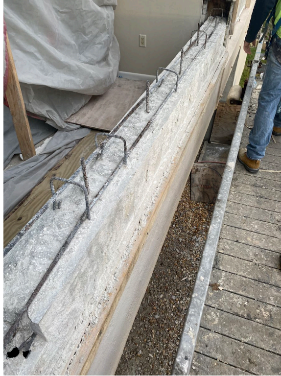
Picture 1: Unit 102 window sill repair
